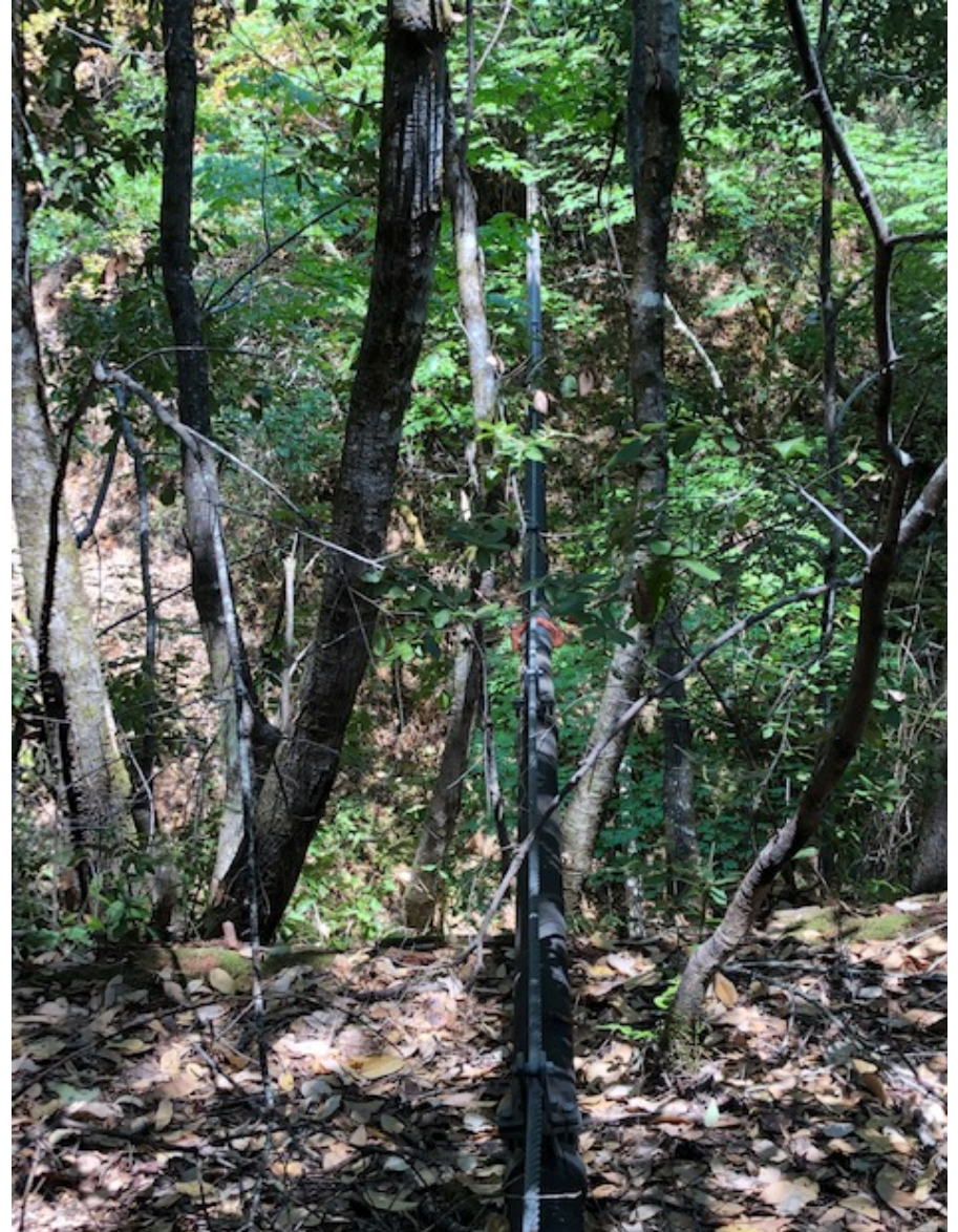
Photo 6. Aerial Sewerline in Gulch from Westerly End
