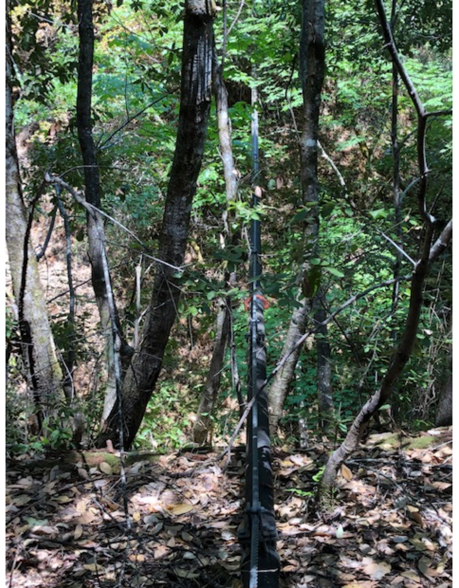
Photo 6. Aerial Sewerline in Gulch from Westerly End
