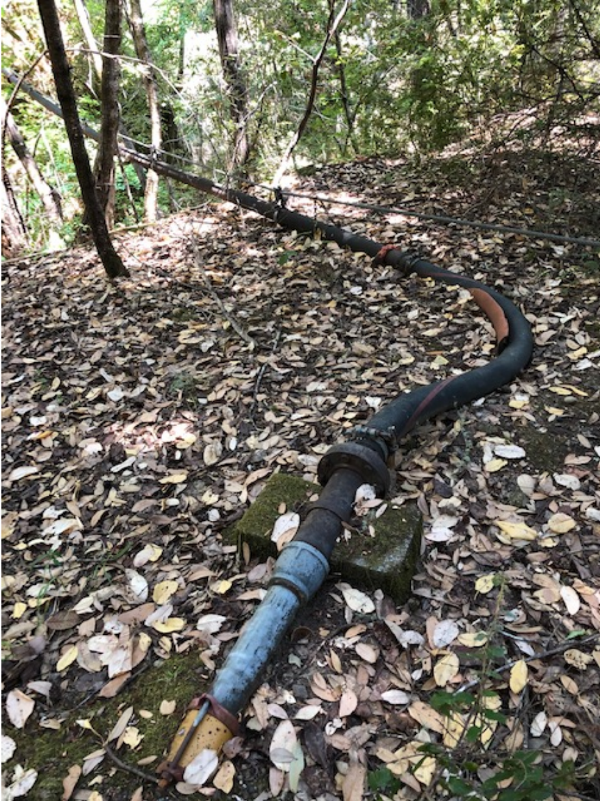
Photo 5. Westerly End of Aerial Sewerline
