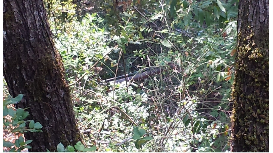
Photo 2. Aerial Sewerline from East Deadman
