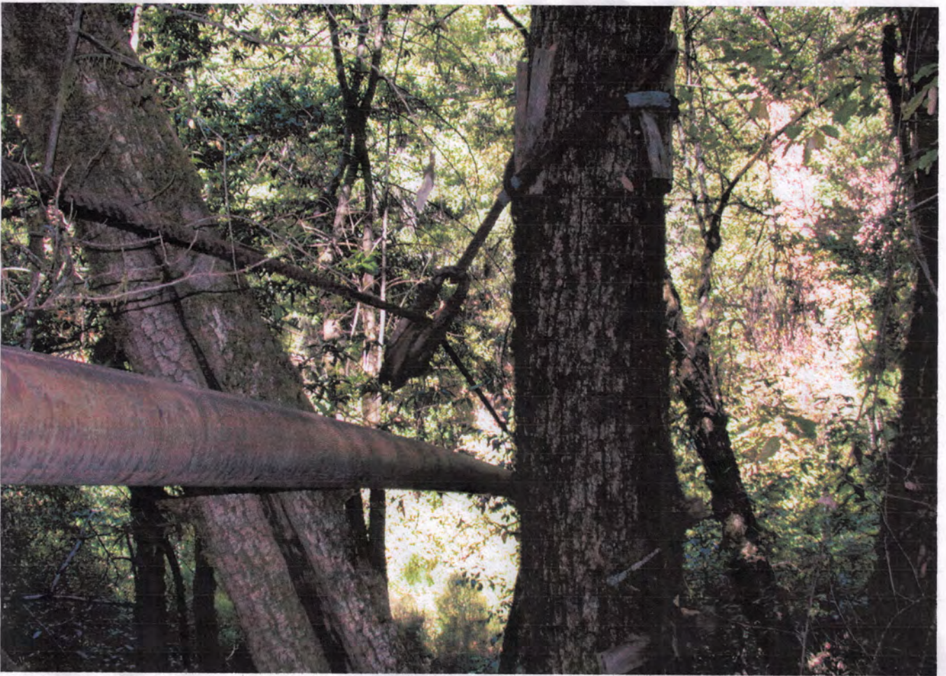
Connection of aerial waterline to trees @ each side of gulch
