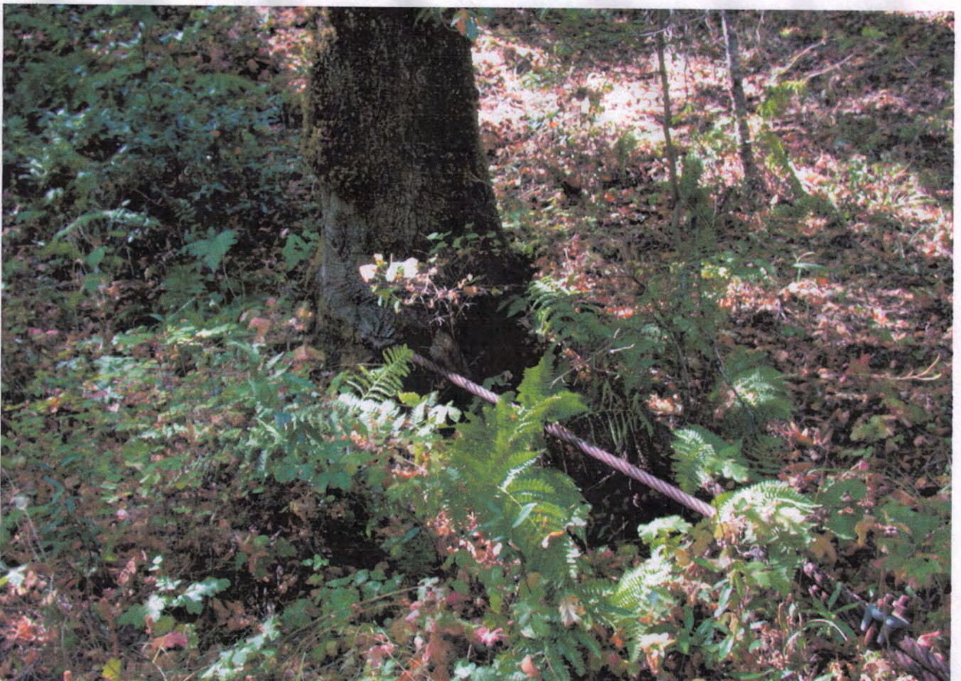
Connection of aerial waterline to trees @ each side of gulch
