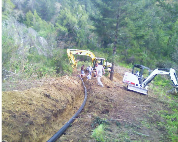
Various photos of the temporary reroute around the landslide area and the connections downsizing the line from 6" to 4" and 3",
