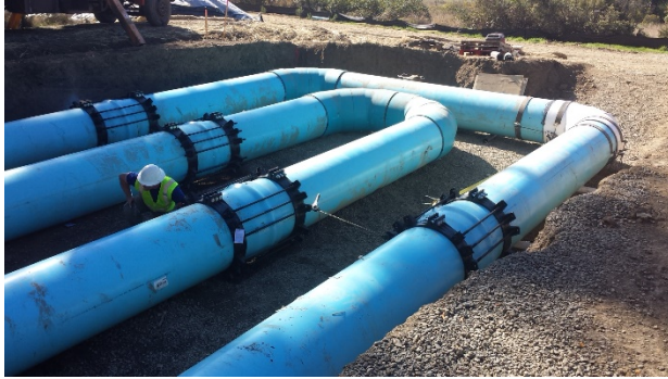
Photo #1 New CT Chamber Prior to Backfill During Construction
