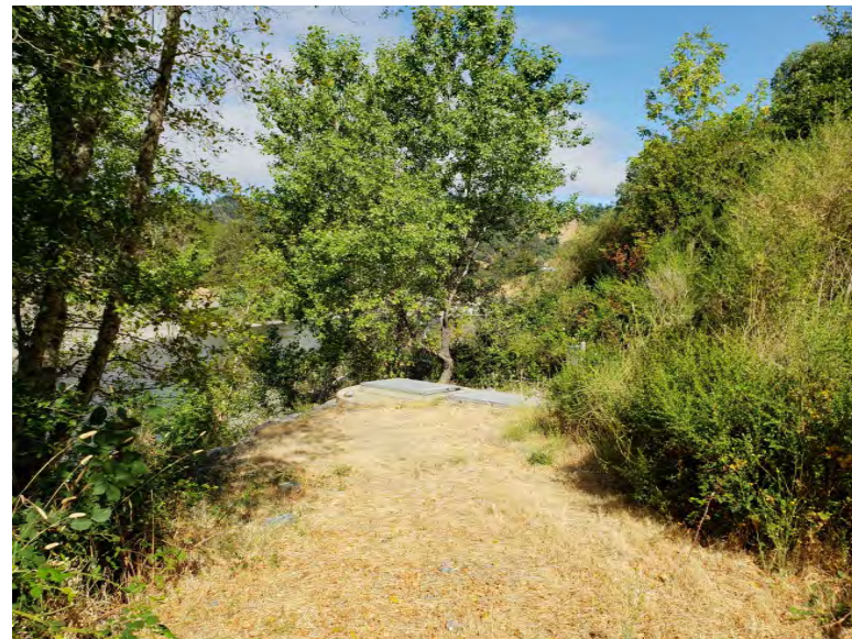
LID OF INTAKE WELL
