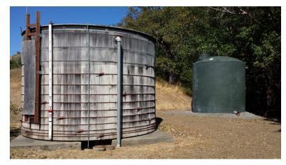
Replacement of the tank with a tank of similar size is likely the long term solution. Utilization of the existing foundation will be considered should it be structurally sufficient and appropriately sized for the new tank. The District holds easements for the existing site and the waterline feeding the tank.
